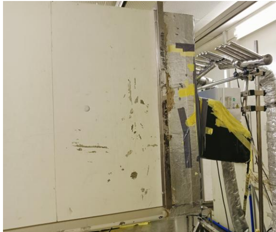
Figure 2. Psychrometric laboratory installation: airflow-rate measurement of the indoor-unit fan
